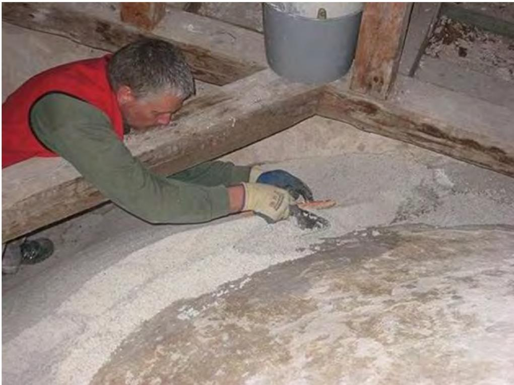
Figure 3. Application of thermal insulation plaster on a medieval church vault (photo: Poul Klens Larsen)
